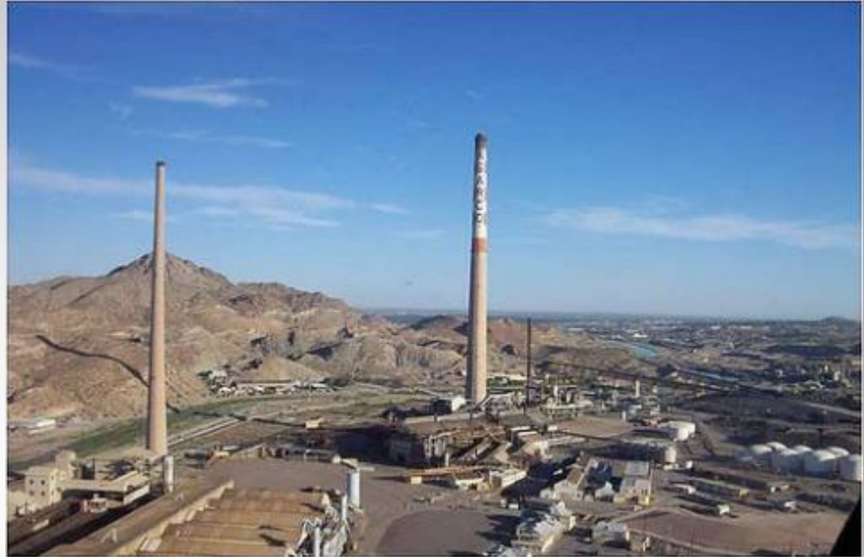
Asarco El Paso: Ores roasted to drive off sulfur and smelted.
